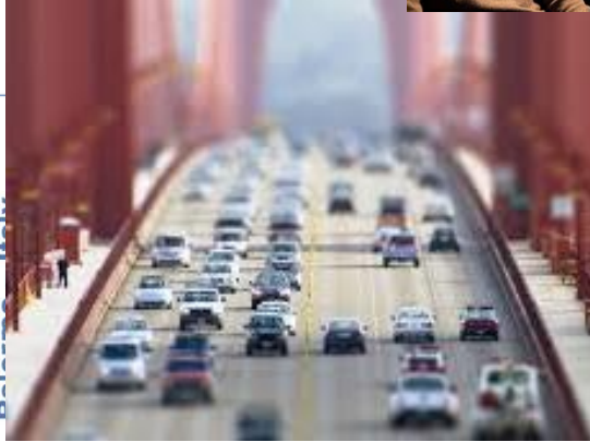
Structure in operating conditions
