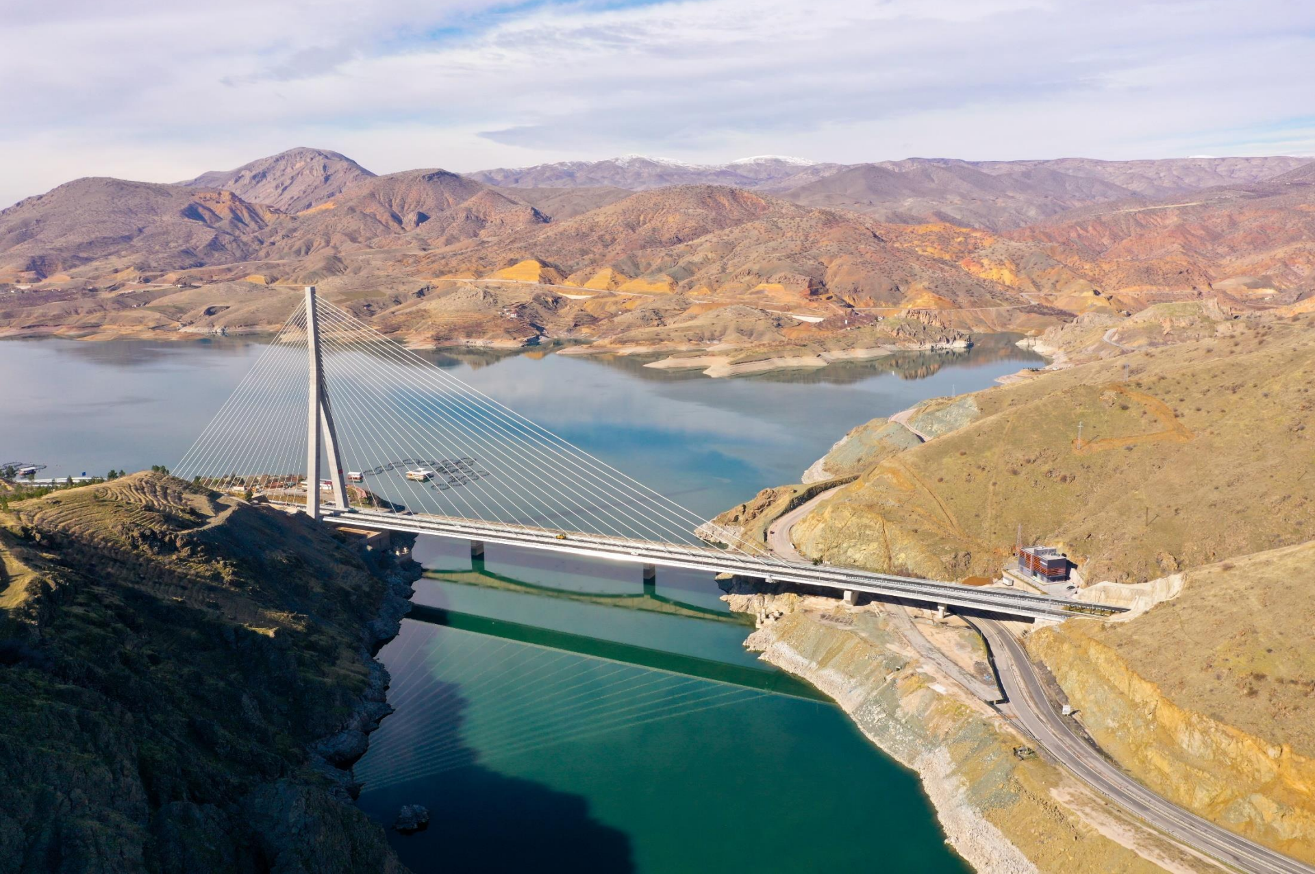
Kormurhan Bridge (380m) 2021-24 Asset Management, Monitoring
