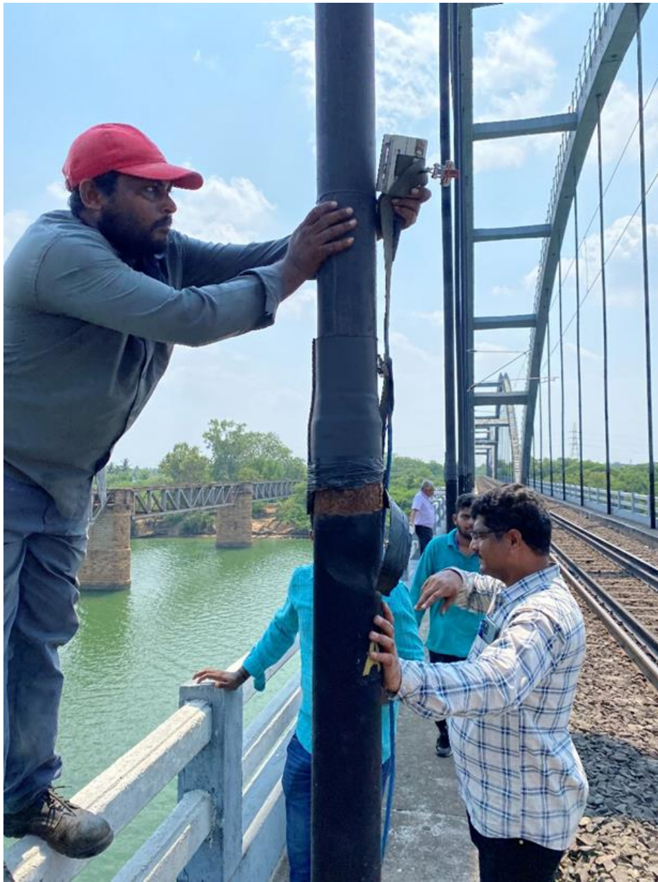
Rajahmundry Railway Bridge (100m) 2023, Condition Monitoring
