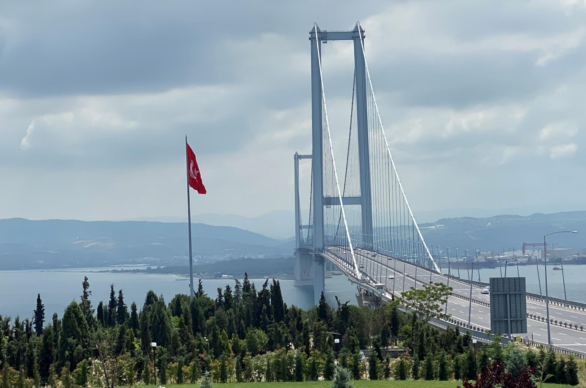
Osmangazi Bridge (1550m) 2012-24 Asset Management, Monitoring
